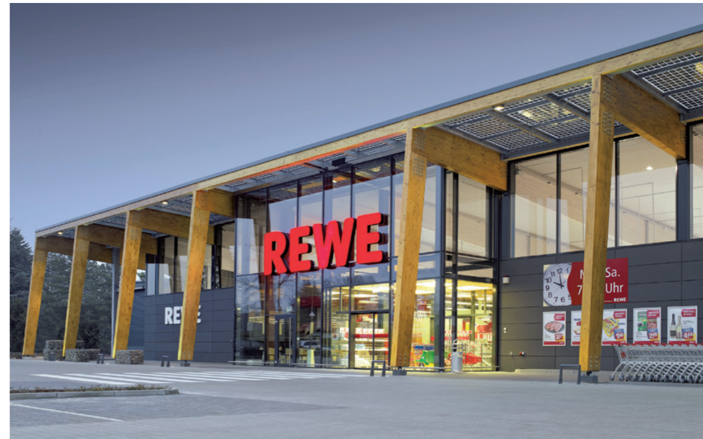
REWE Green Building
